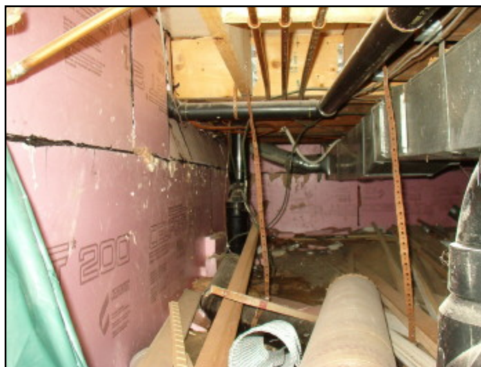
13. Exposed polystyrene insulation is fire hazard
