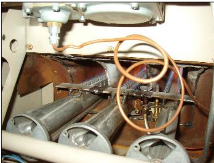
9. Rust at bottom of heat exchanger
