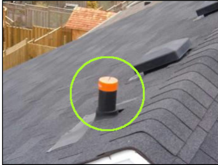
16. Plumbing stack is capped
