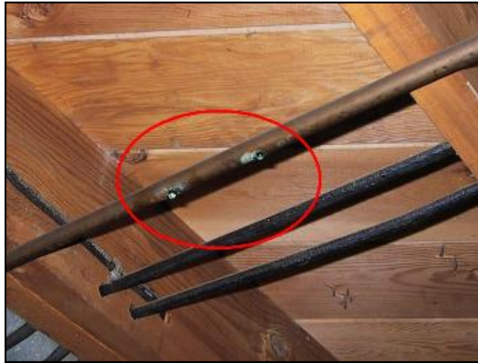
14. Leaking copper supply pipe
