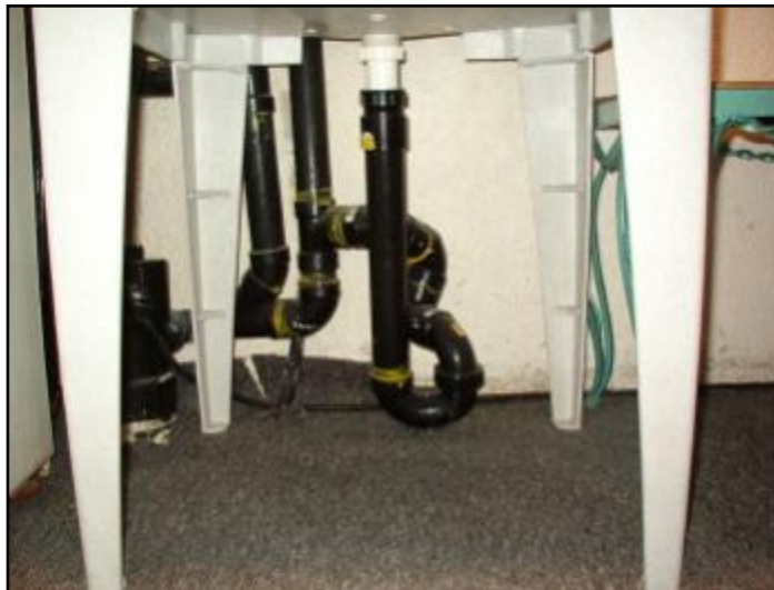
15. Poor trap arrangement
