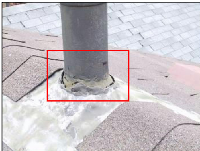
2. Stack flashing should be sealed.
