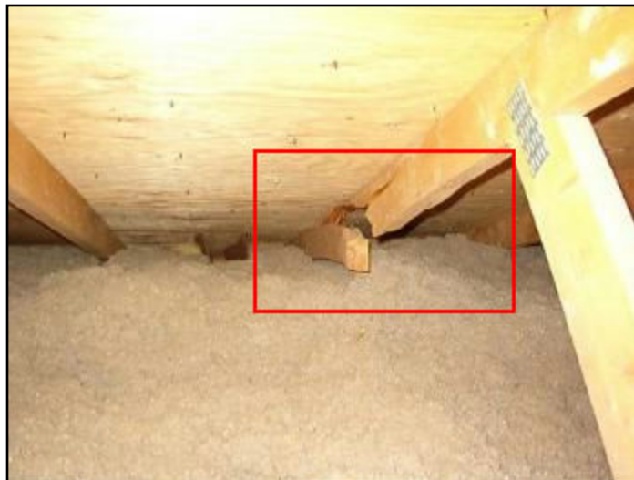
5. Top chord of truss is broken
