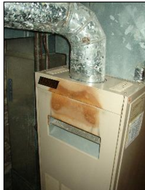
10. Evidence of furnace backdrafting
