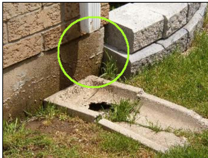
3. Downspout should be extended away from home
