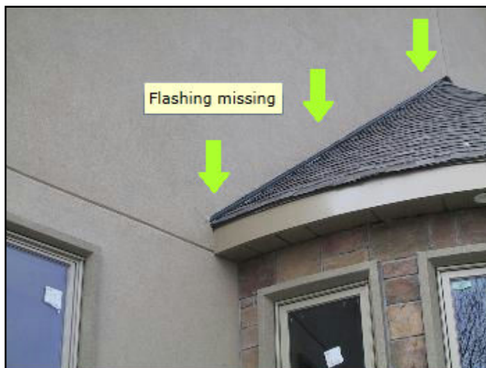
1. No kickout flashing at roof/sidewall junction
