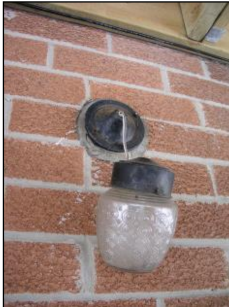
7. Light fixture is not well secured
